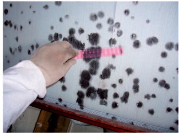
Fig. 4. Contact sampling of molds on walls.
