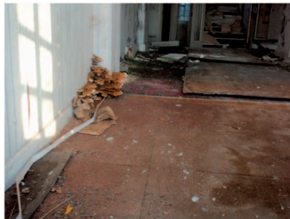
Fig. 2. Dry rot fruiting body and spores.
